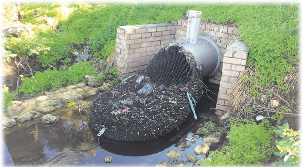
Figure 2 Kiwanawa implantation of drainage nets successfully captures 370kg's of rubbish waste (Utarait, 2018)
